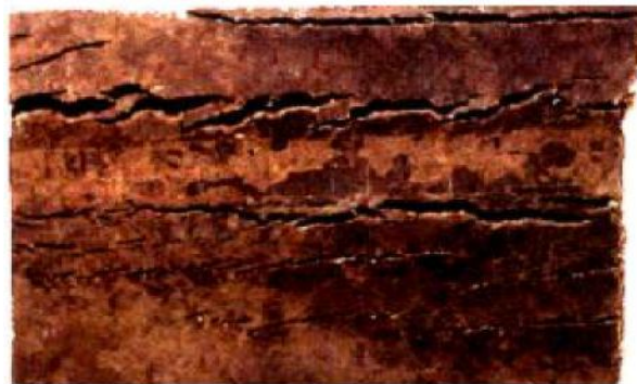
Figure I.5 Fissures de CSC [5].
