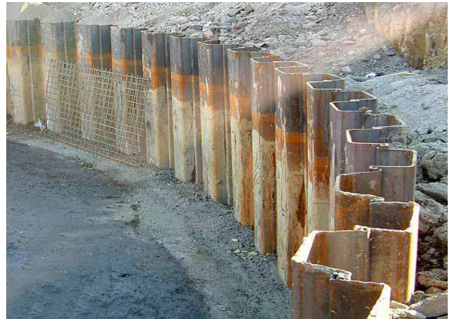
Figure I.8: Rideau de palplanches.
