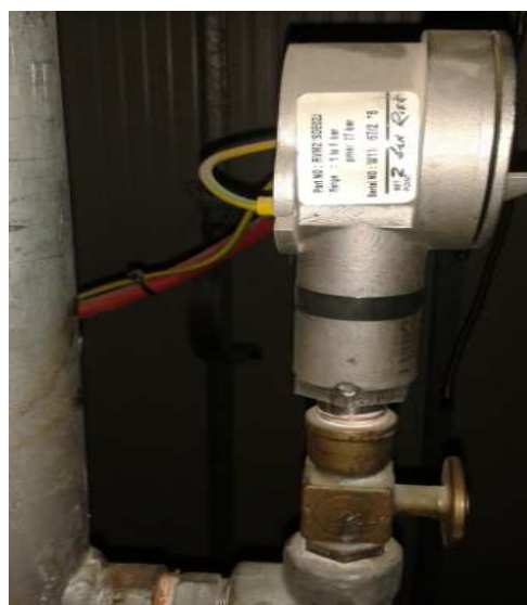
Figure II.13 : pressostat.
