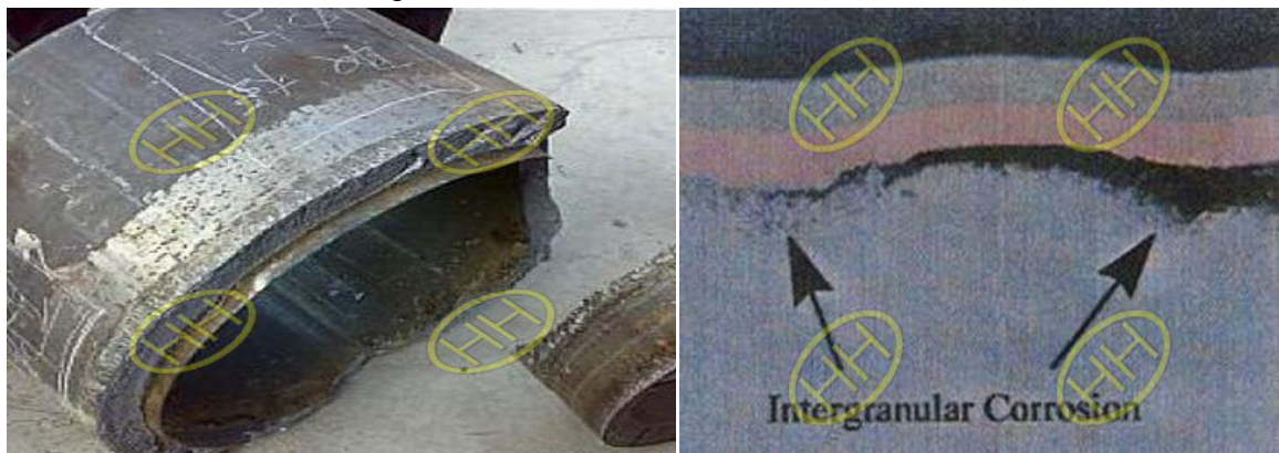
Figure 1.5 corrosion inter granulaire [7]
