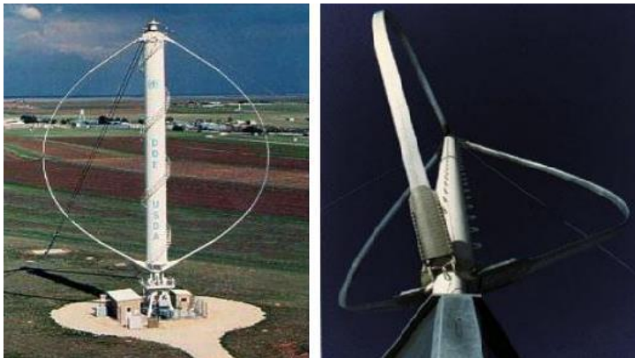
Figure I- 10: Darrieus "eggbeater" turbine
