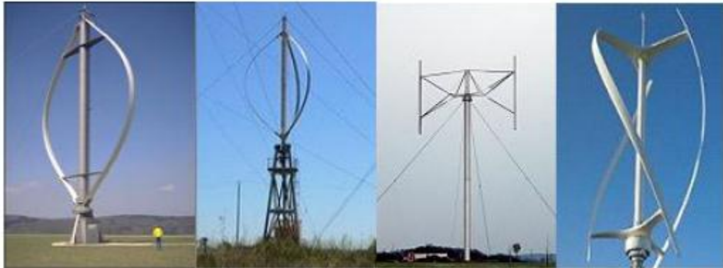
Figure I. 3: Vertical axis wind turbine (VAWT)
