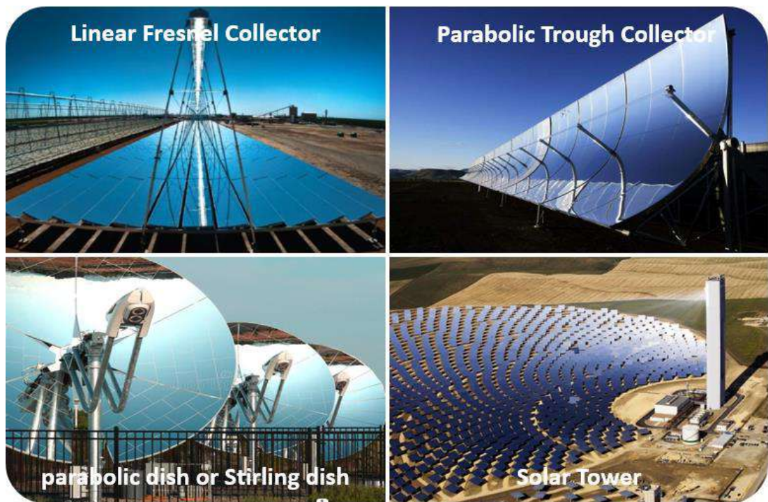
Figure 1.2: Concentrated Solair powerr (CSP) technologies.
