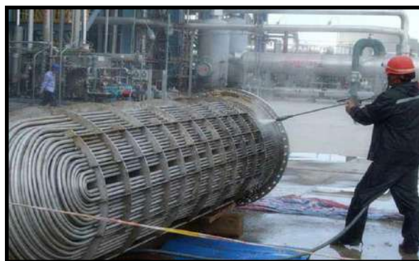
Figure 3 Manuel heat exchanger cleaning [1]
