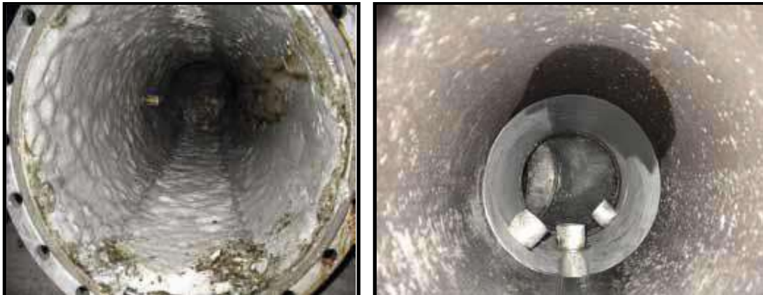
Figure 5 Pipe cleaning operation [1]
