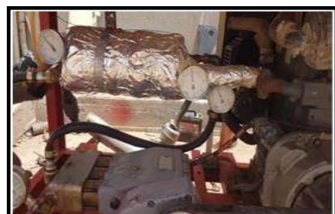
Figure 49 Exchanger isolation and final installation
