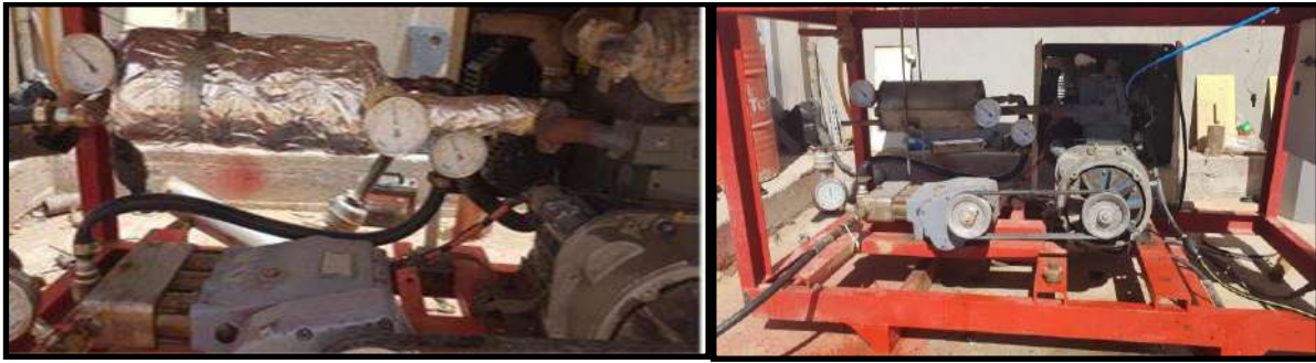
Figure 51 The final skid installation
