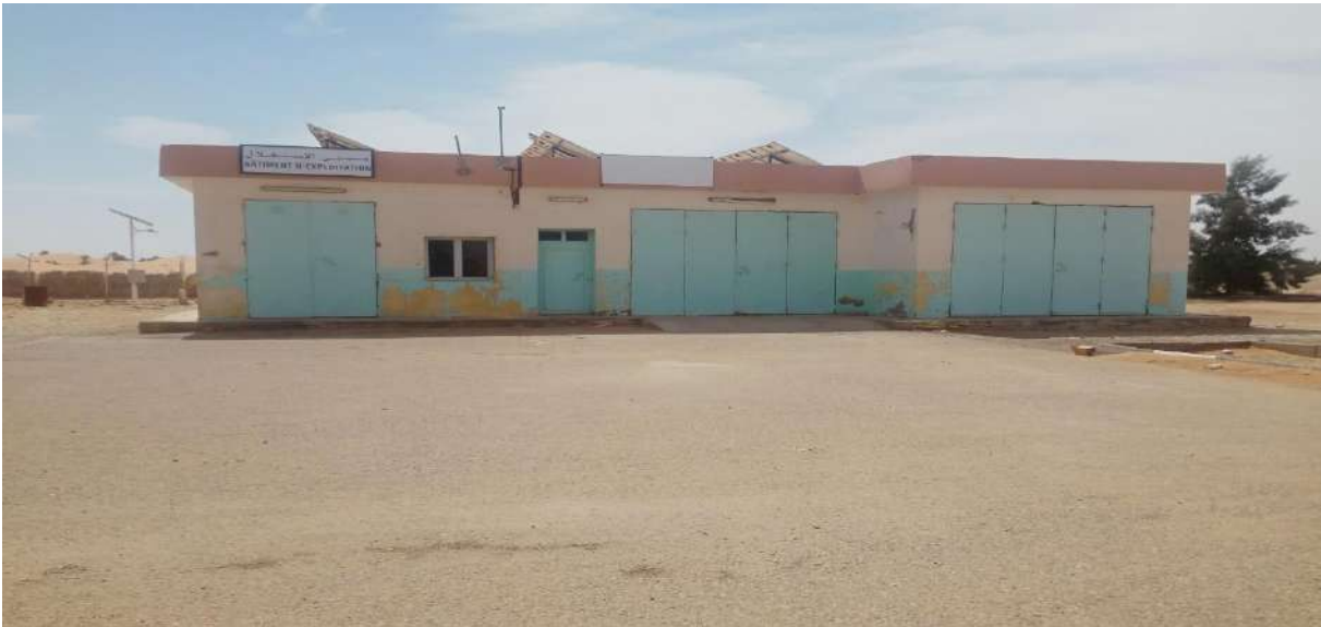
Figure II.3: Station d'épuration de sidi khouiled
