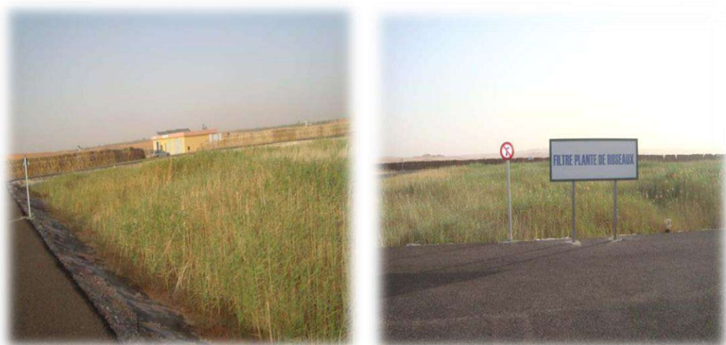
Figure II.15: Filtre planté roseaux
