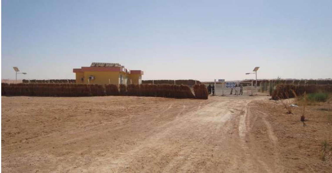
Figure II.4: Station d'épuration de N'goussa
