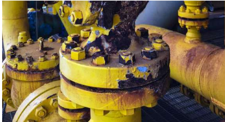
Figure I.5: crevice corrosion [6]
