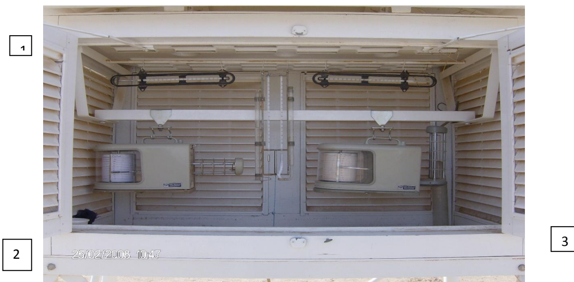
Figure15: Weather shelter (Photo taken by students).
