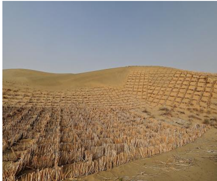
Figure I-5: Reed checkerboard barriers
