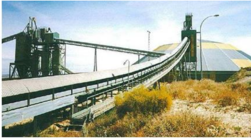
Figure II-1: General view of the conveyor belt
