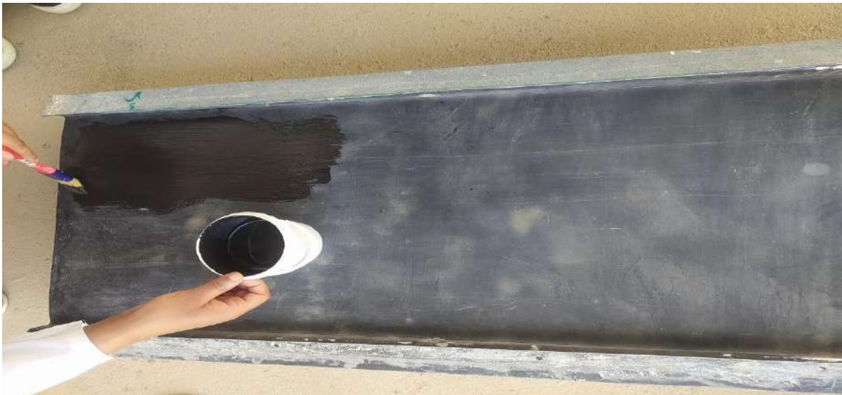
Figure (III.33) Painting the absorber process
