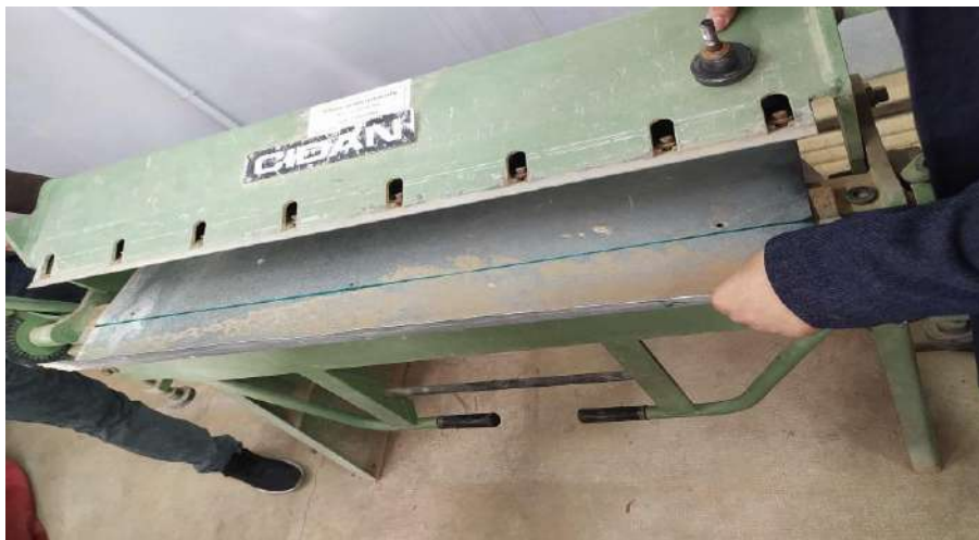
Figure (III.9) Banding the steel sheets
