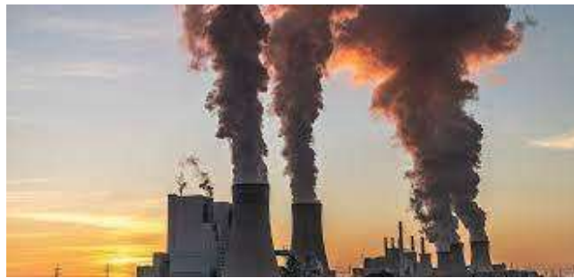
Figure II.2. Centrale au charbon
