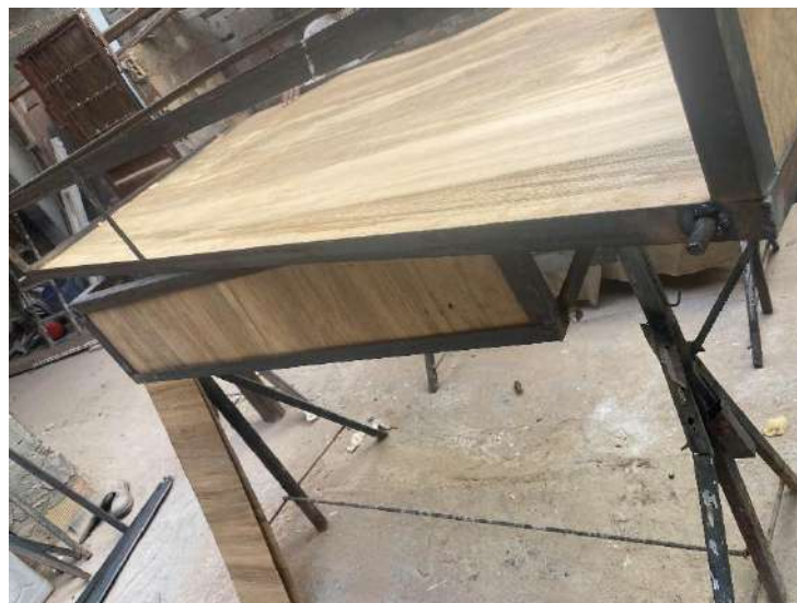
Figure (3- 1): Construction of the box
