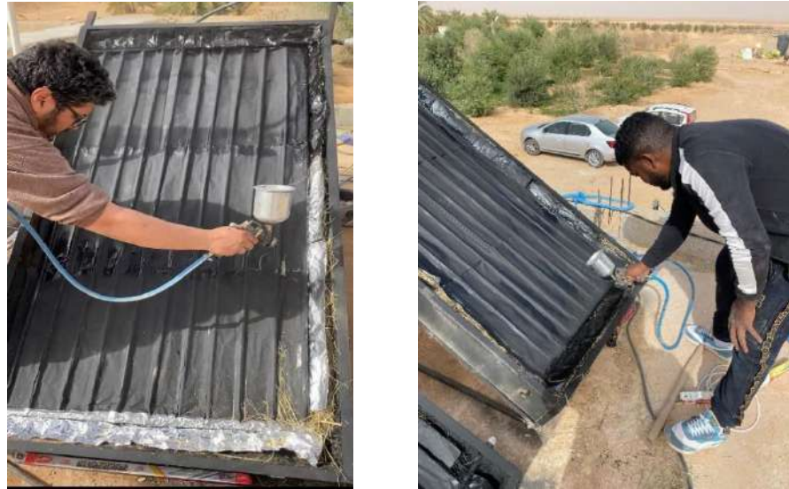
Figure (3-3): Dyeing aluminum sheets
