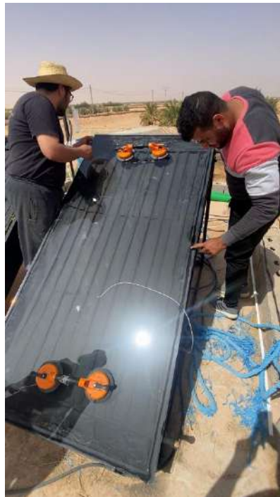
Figure (3-4) : Glass Installation Process
