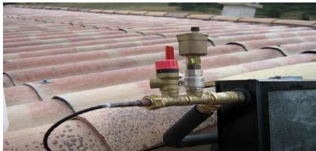
Figure (1-9): Drain valve
