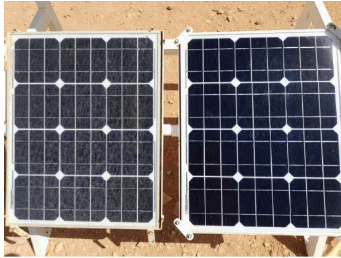
Figure (III-41): Experimentation facility (11/05/2022).
