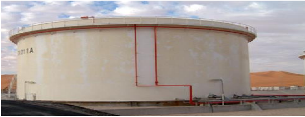
Figure I- 10 :storage tank TK 211 [02]
