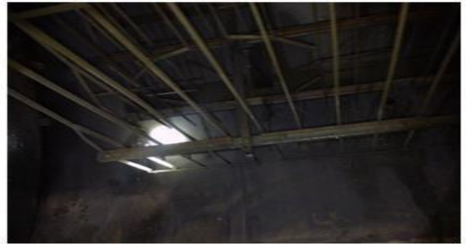
Fig.III..3:The horizontal grids in side Desalted (V-103 left,V-104 right)
