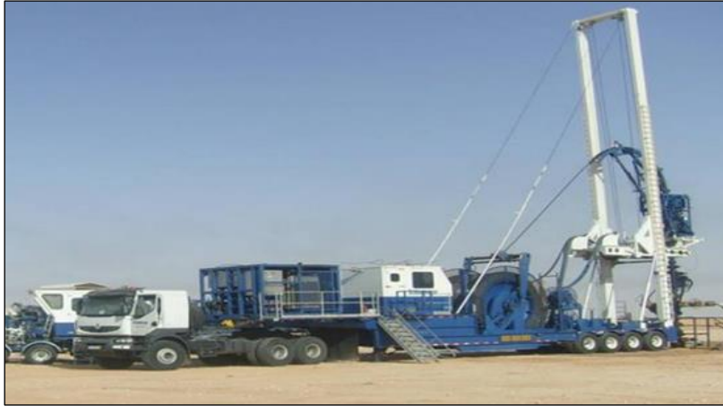
Figure. III.9: Opération Coiled tubing
