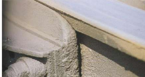
Figure I.41. Stock Rail Headwear Associated with a Used Switch Rail
