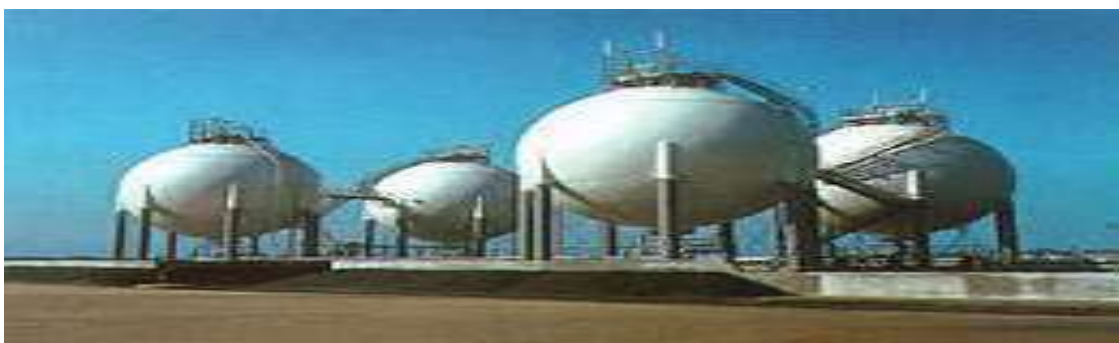
Figure 7 LPG spherical storage [16]
