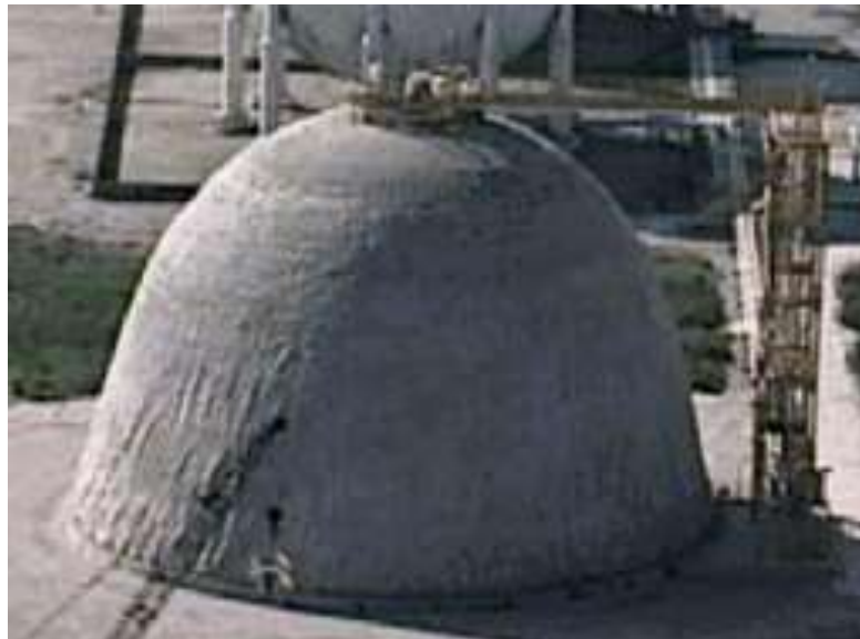
Figure 9 LPG storage tank under bank [16]
