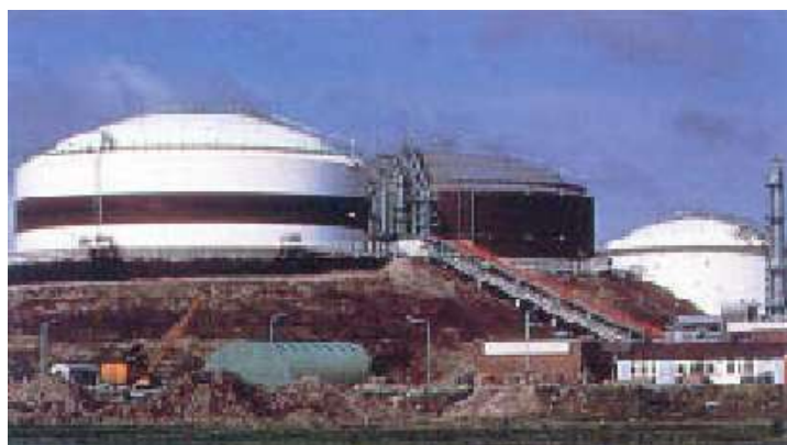
Figure 10 LPG refrigerated storage [16]
