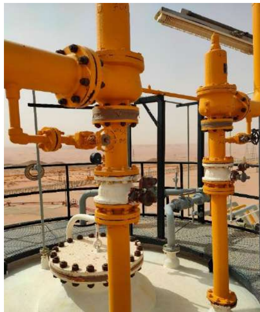
Figure 28 PSV above the sphere
