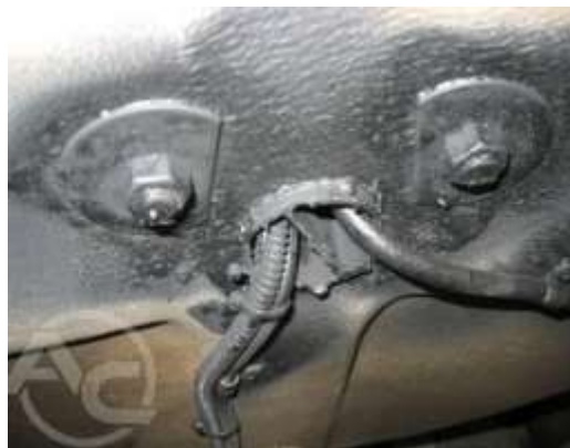
Figure II.4: The view from underneath of the vehicle after installation of the tank [12].
