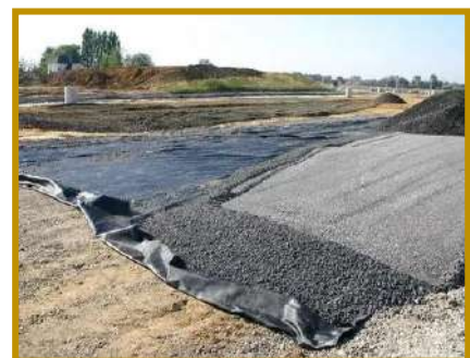
Figure 1.8: Geotextiles for reinforcement.
