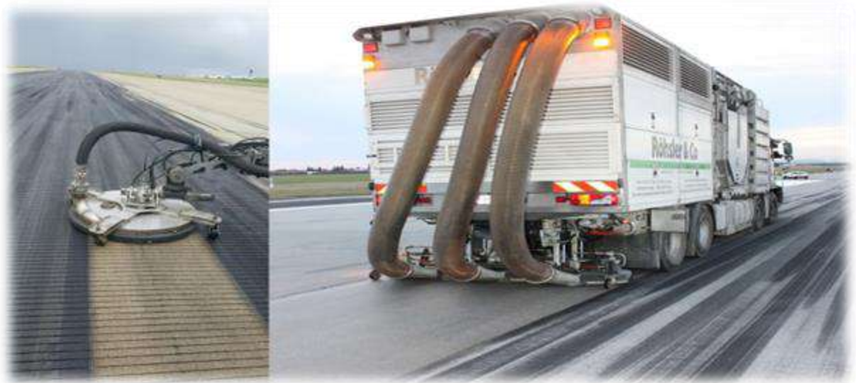
Figure (III.01): A device for removing the rubber layer with chemicals or hot water
