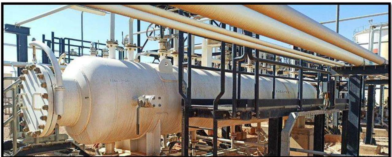
**Figure II.8 Induced Gas Flotator (IGF)**
