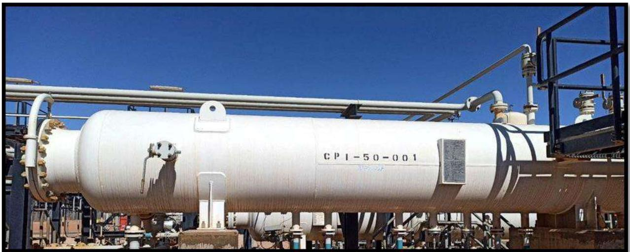
**Figure II.7 Corrugated Plate Interceptor (CPI)**
