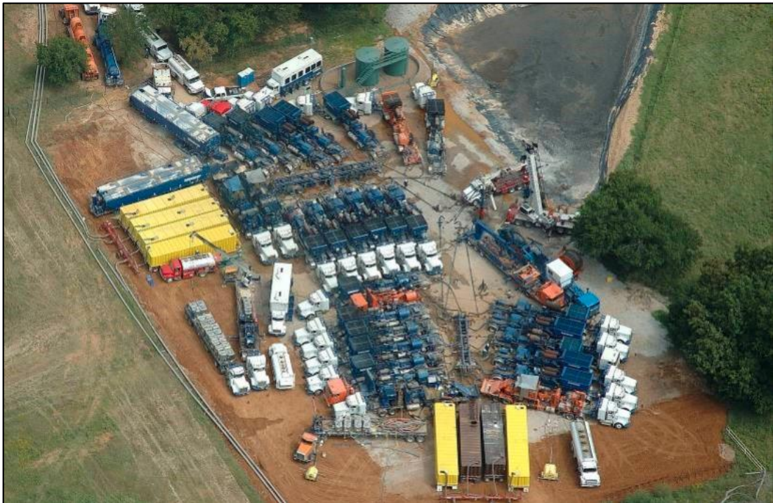
Figure I.4: Hydraulic fracturing equipment.[10]
