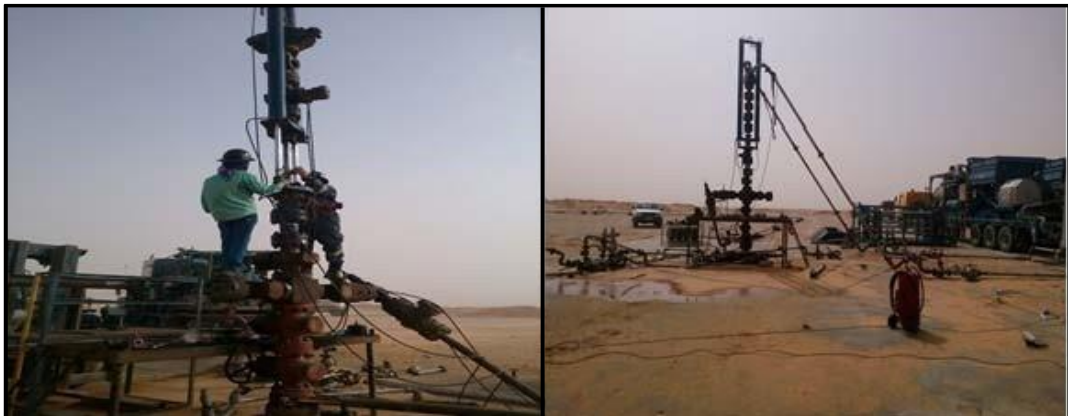
Figure II.20 : Montage du 'Tree Saver'
