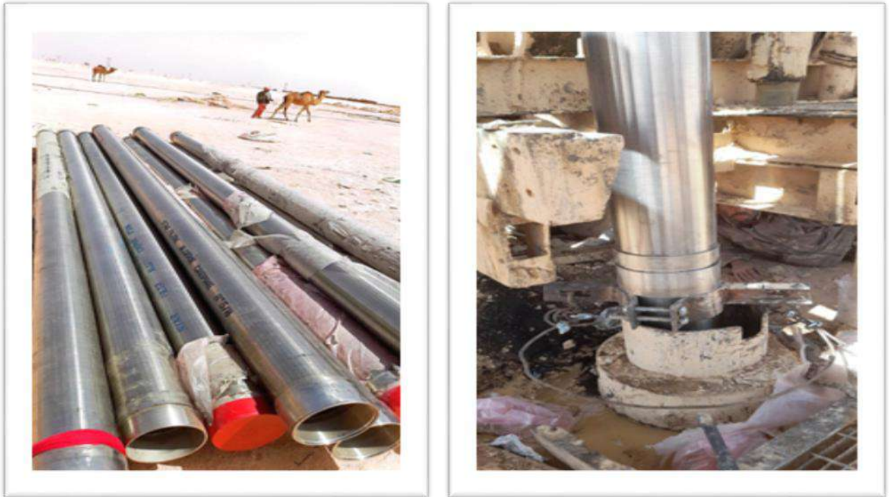
Photo 20: tubes de crépine Johnson
