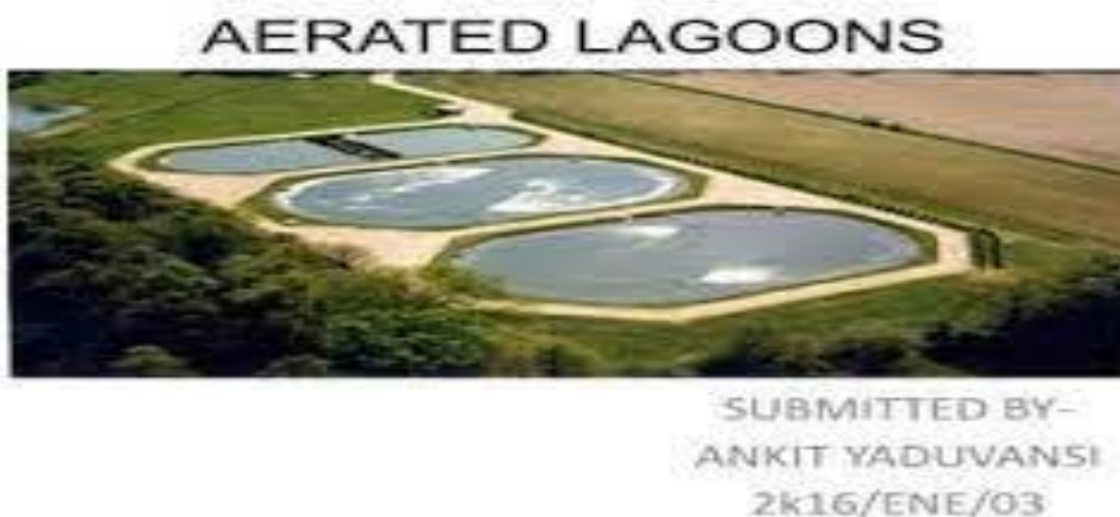
Fig (II. 10): Aerated lagoon
