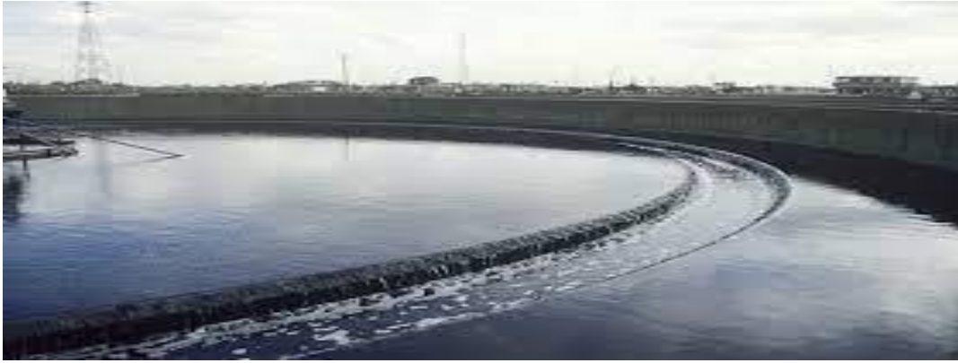
Fig (II. 12): Secondary settling.
