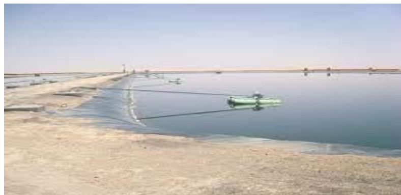
Fig (III. 9): Aeration lagoon in the Ouargla station.
