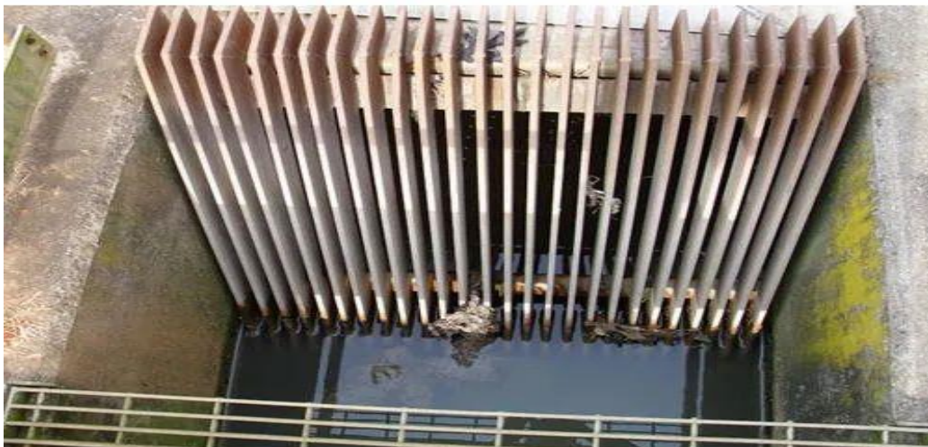
Fig (III. 6): Screen in the Ouargla station.
