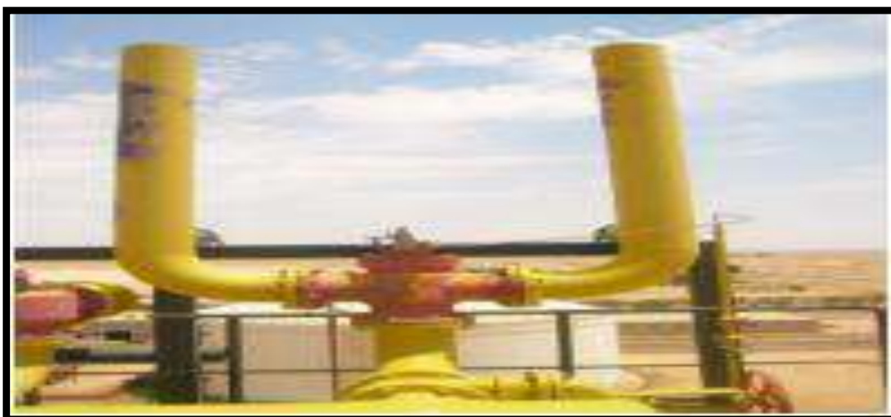
Figure I4. – Safety valve
