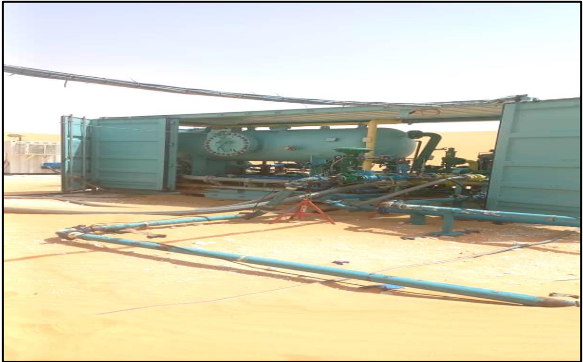
Fig III.2: Separation section (11 May 2024)
