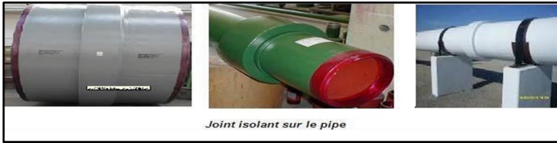
Figure II.5: Insulating joints.[9]
