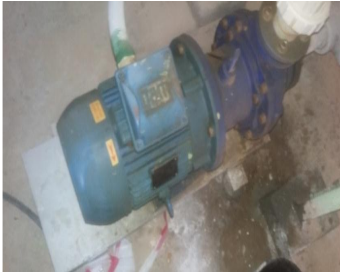
Figure II.8 : La pompe centrifuge
