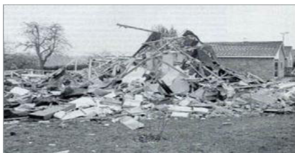
Figure.3. A house destroyed by methane explosion at Loscoe, Derbyshire
