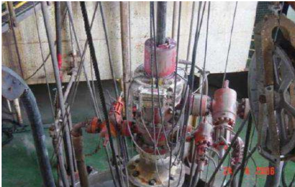
Figure 7 Subsea RCD (SSRCD) installation in moon pool 25
