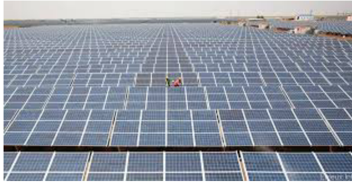
Figure I-17 : Centrales solaire photovoltaïque de Kamuthi (India)
