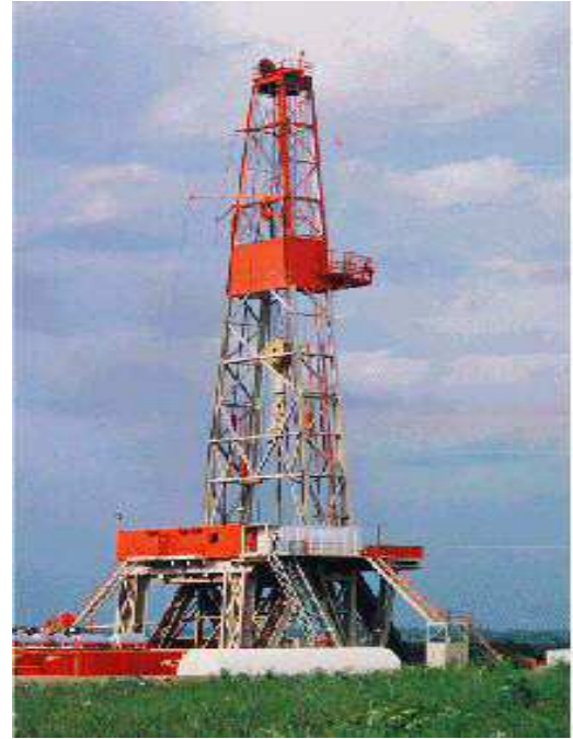
Figure II.3: Mâts de work over
