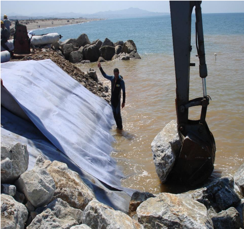
Station Dessalement Alger
