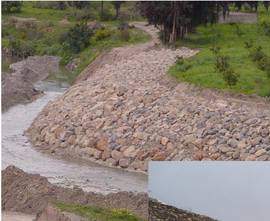
Autoroute Est/Ouest Oued Djer
