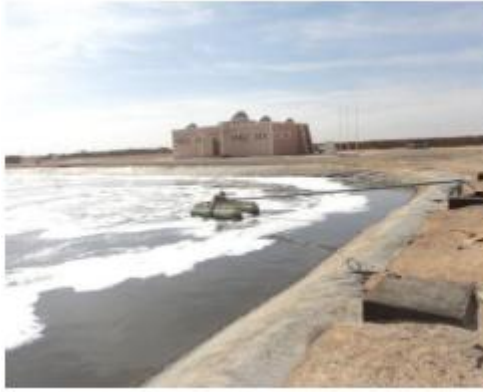
Figure (III-11): Lagune aéré
