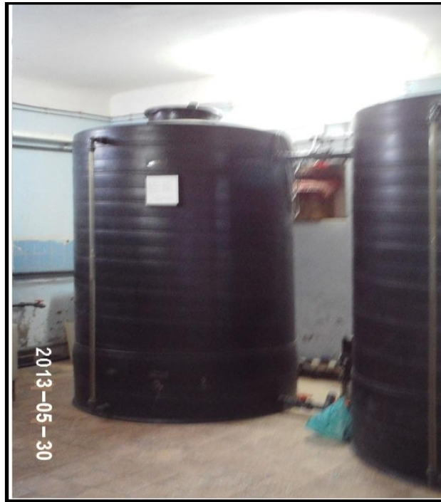
Photo-05 : cuves de stockage eau potable
