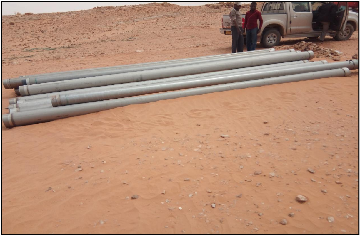
Crépine Inox type Johnson (slot 20, \text{Ø}8^{5/8} " )
