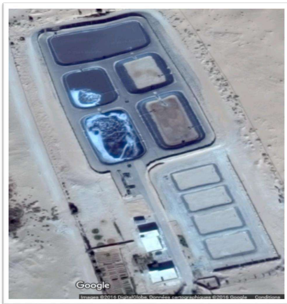
Photo 08: la station d'épuration de sidi khouiled (Maps. Google201
