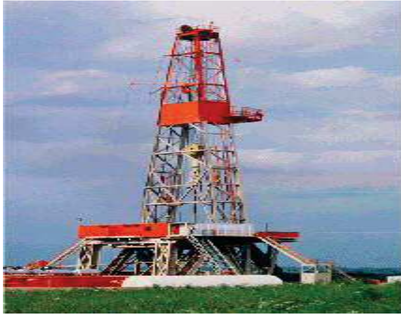
Figure 8:mât de forage. [13]
