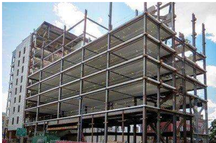
Figure II-1 : Construction of Steel Frame Structure
