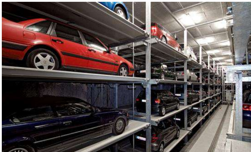
Figure I-12 : View into one of the two parking shelf systems
