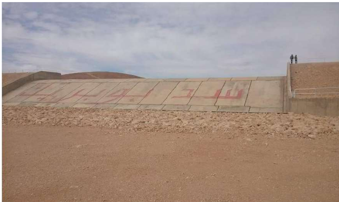
Figure II.11: Photo du Barrage Bou Brik [NESRAT.D ; ZINALO ,2018]
