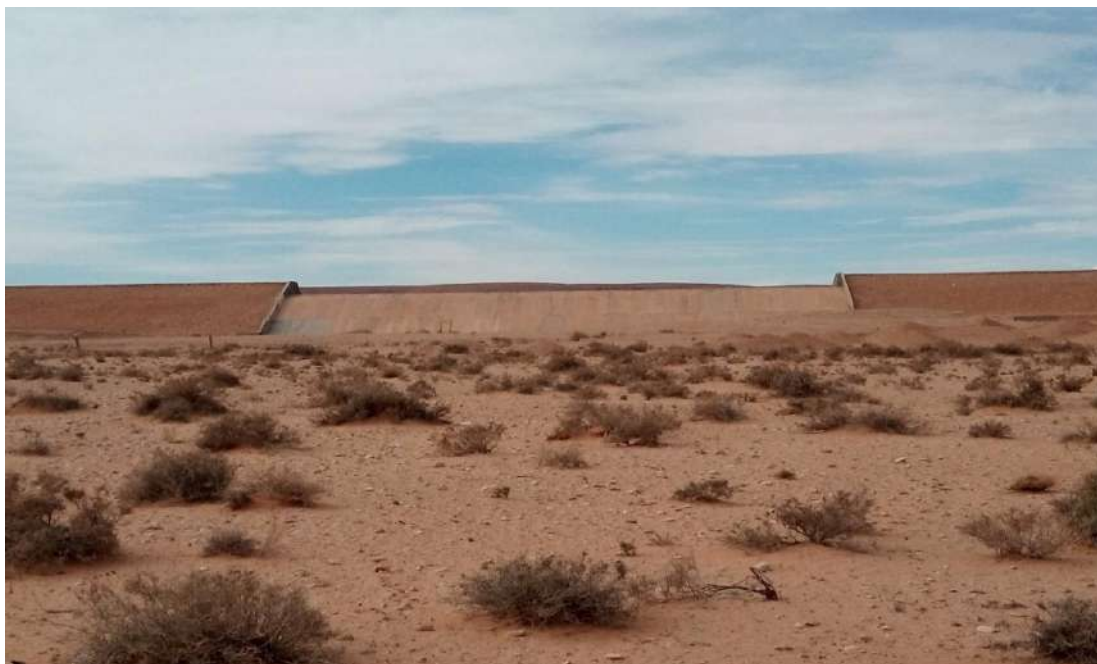
Figure II.12: Photo du Barrage El Abiod[NESRAT.D ; ZINAIO ,2018]
