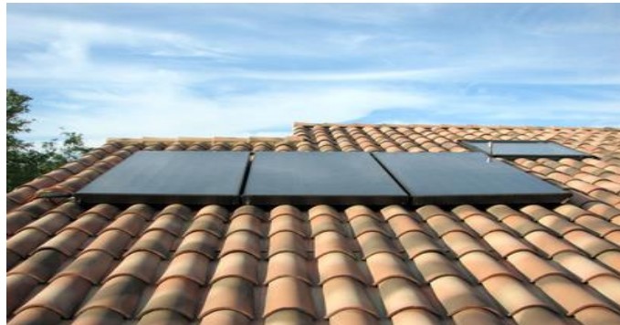
Figure 27: Chauffe-eau à circulation forcée
