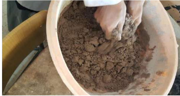
Figure III.3 malaxage manuelle
