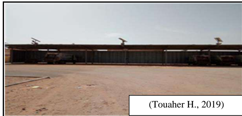
Photo 18: Abri des engins
