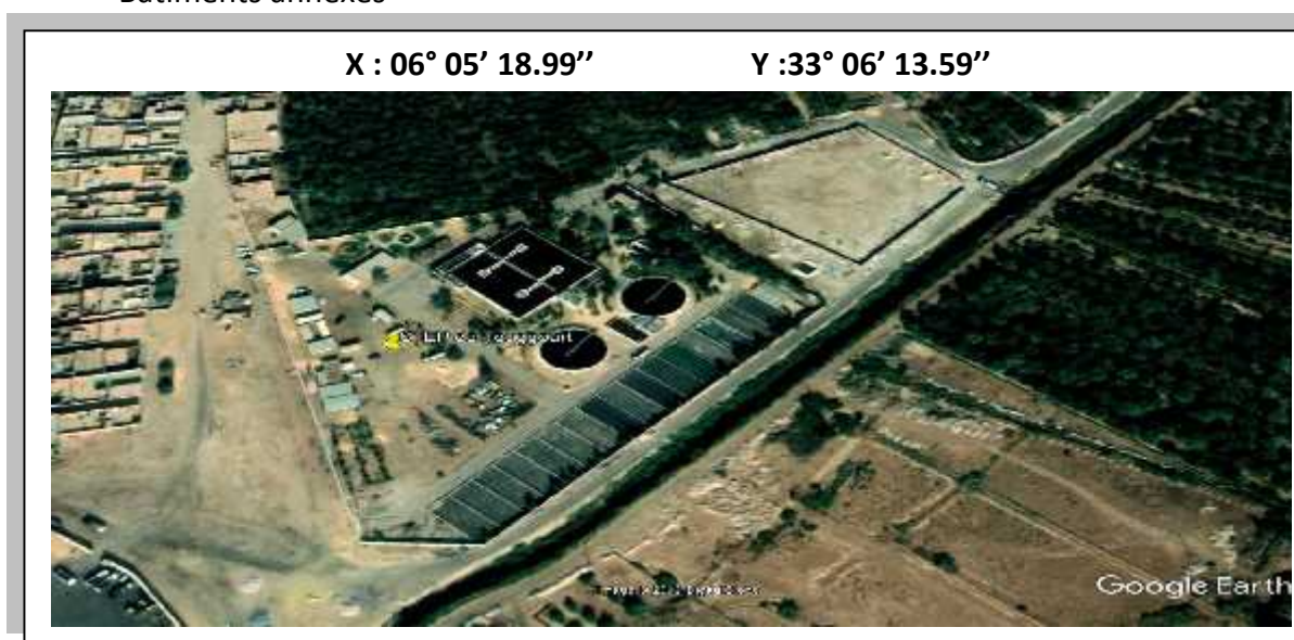
Figure 3- 2: Station d'épuration de Touggourt (Google Earth)
