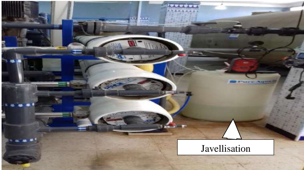
Figure .11. Javellisation (station Sarl Ben Amor).
