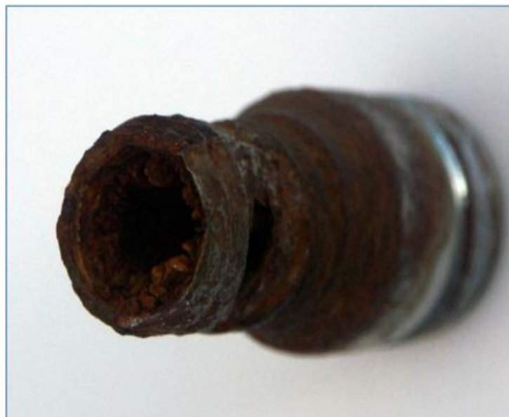
Figure I.6. La corrosion érosion.
